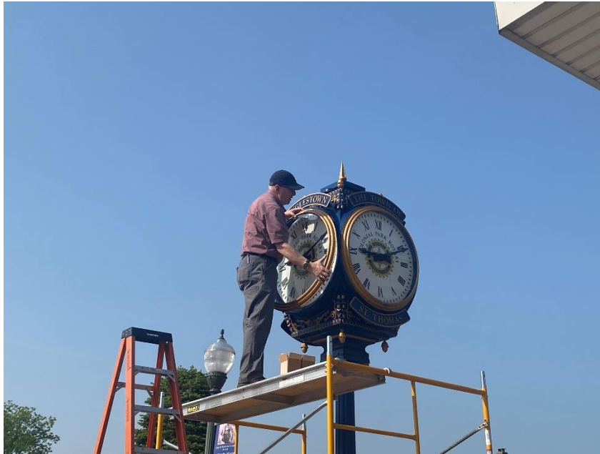
Master clock repairman Bob Rodgers fixes one of the Lingletown Square Clock's mechanisms and performs preventative maintenance to keep it ticking for years.
